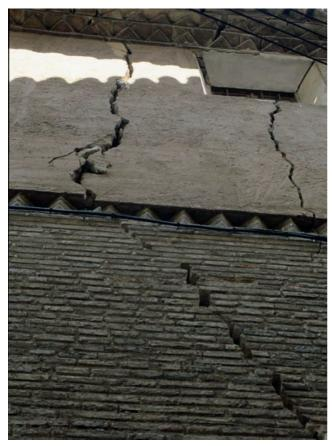
**Fig. 5.** Cracks in historic building of Colegiata Sta. María La Mayor in Calatayud, Spain. Here the cracks are up to 30 mm wide; others on the building are larger and the degree of damage merits a category 5 classification (Gutiérrez & Cooper 2002).
