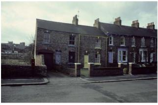
**Fig. 3.** Sagging building damage category 5 caused by gypsum dissolution and associated settlement on peat deposits, Princess Road, Ripon (Cooper 1998).
