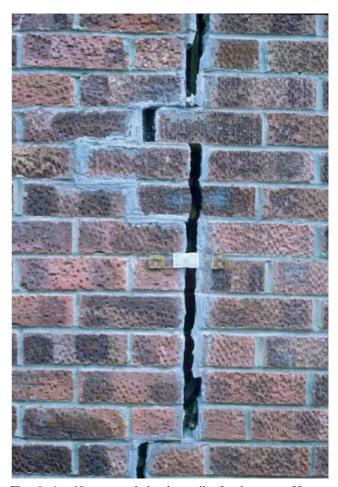
**Fig. 6.** An 18 mm crack in the wall of a house at Hutton Conyers near Ripon; damage caused by subsidence at the side of a large doline formed by the dissolution of gypsum. Category 4 damage formed by loss of support and rotation of the floor slab.
