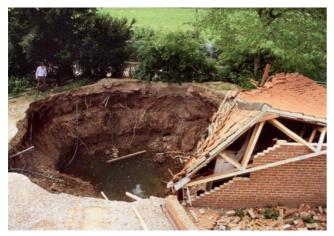
**Fig. 2.** Category 7 building damage at Ure Bank Terrace, Ripon. The damage here has been caused by gypsum dissolution and collapse with loss of support under most of the building (Cooper 1998).
